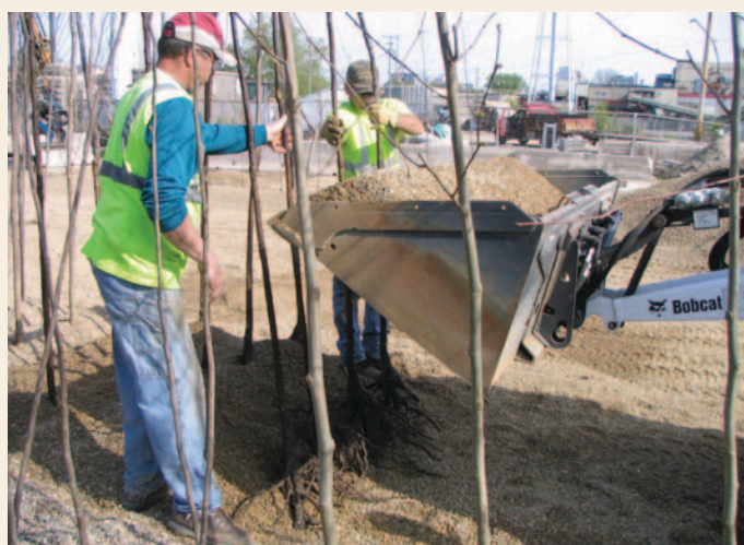
Figure 12. Installing trees with a machine in Rochester, MN
